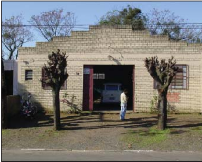
FRONT OF BUILDING
